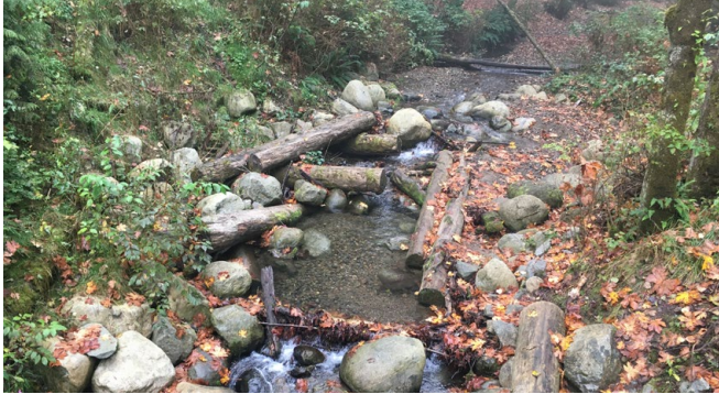
Figure 12: Instream structures constructed with woody debris. Source: City of Surrey, BC.
