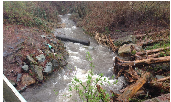
Figure 11: Photograph of a woody deflector in a channel. Source: City of Surrey, BC (a). Schematic of a woody deflector in a channel (b).
