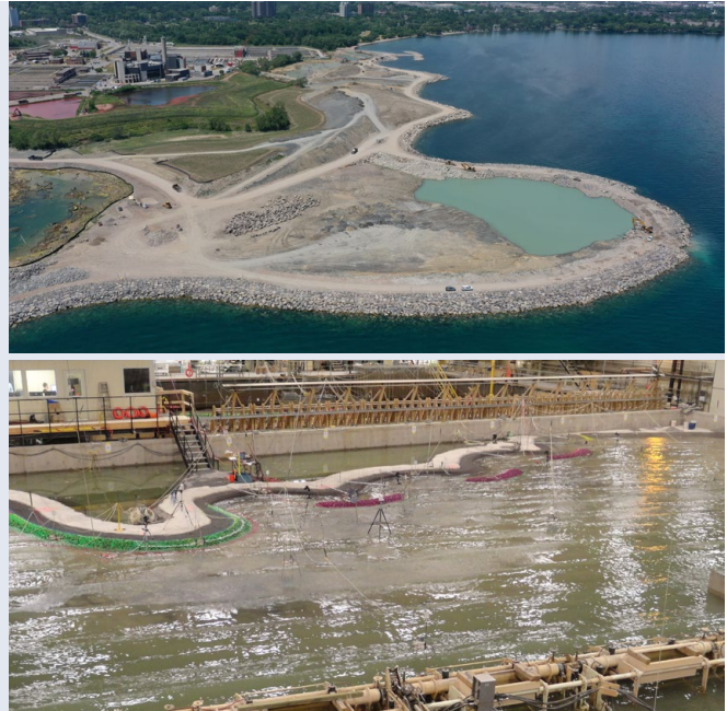
Figure 7: Lakeview waterfront restoration (a), Source: The Region of Peel, Credit Valley Conservation and Toronto Region Conservation Authority; Physical model of Lakeview waterfront at National Research Council Canada's research facilities, Ottawa (b), Source: National Research Council Canada.
