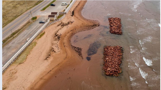
Figure 9: NbS for coastal erosion at Souris. Reproduced with permission from M. Davies, Coldwater Consulting Ltd.
