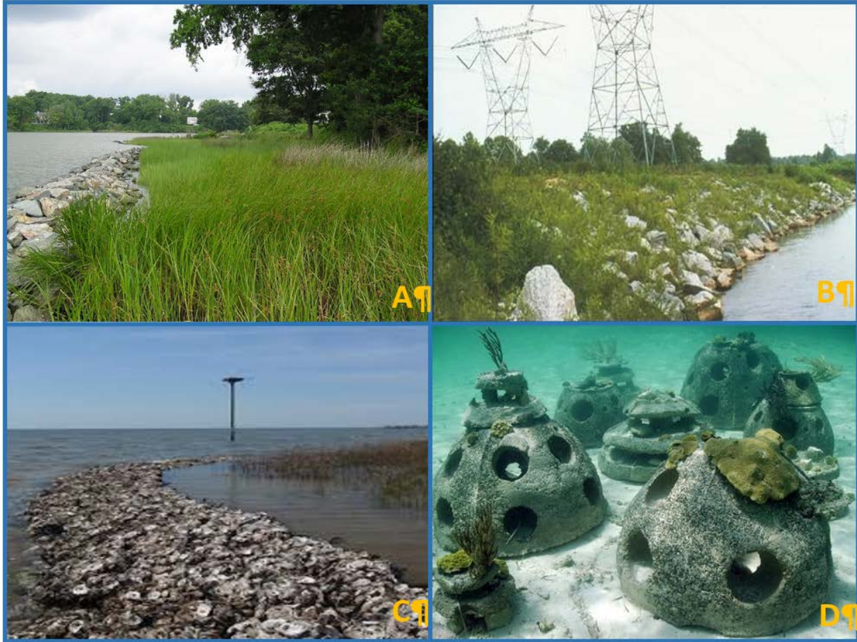
Figure 1: Example Living Shorelines Projects (A - Marsh Sill, B - Joint Planted Revetment, C - Oyster Reef, D - Reef Balls)
