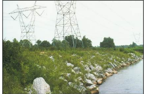
Figure 8: Typical Joint Planted Revetment
